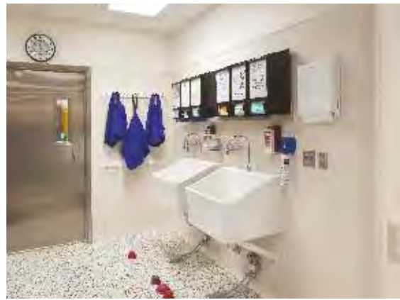
Hospital Scrubs Sinks made with DuPont™ Corian®, East Texas Medical Center, photo DuPont™ Corian®, all rights reserved.
